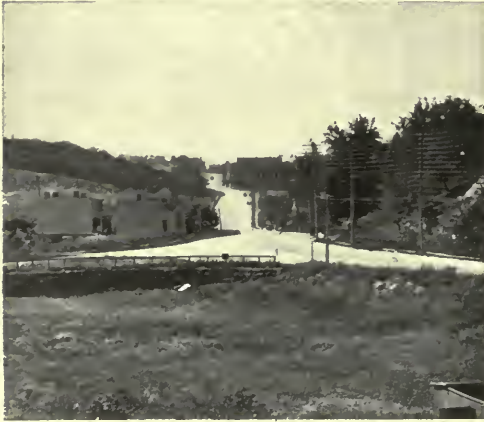
Kingsbridge Road, N. Y. C., Looking South. The ugliness of successive angles in a road that should have been made in natural curves.
